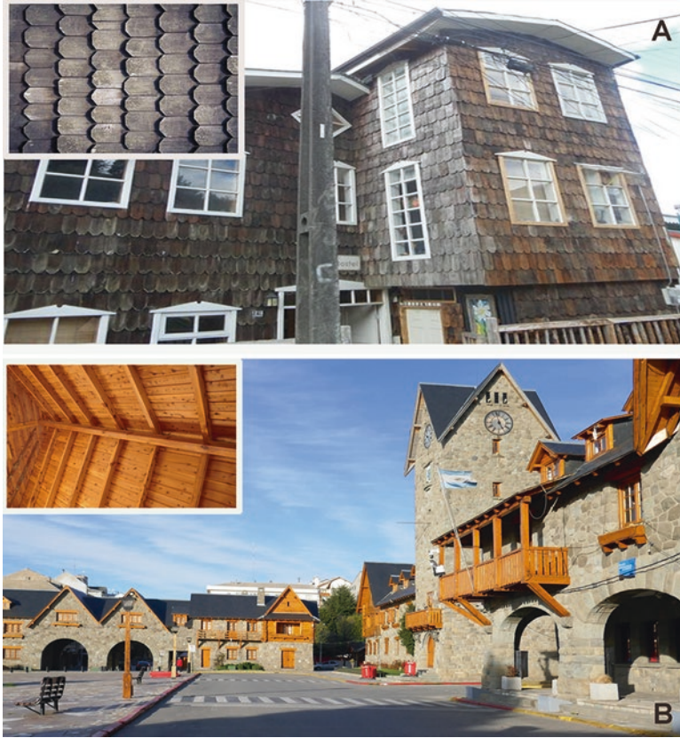
Fig. 2.3 Buildings made with native species. (a) Typical house in the south of Chile made with Fitzroya cupressoides tills (see inset with details of the tills). (b) “Centro Cívico” of Bariloche, Argentina, where the city council functions, made with wood of Austrocedrus chilensis , and closer look to a roof in the inset. (Photos a downloaded from www.tripadvisor.com , b by L. Gallo)
