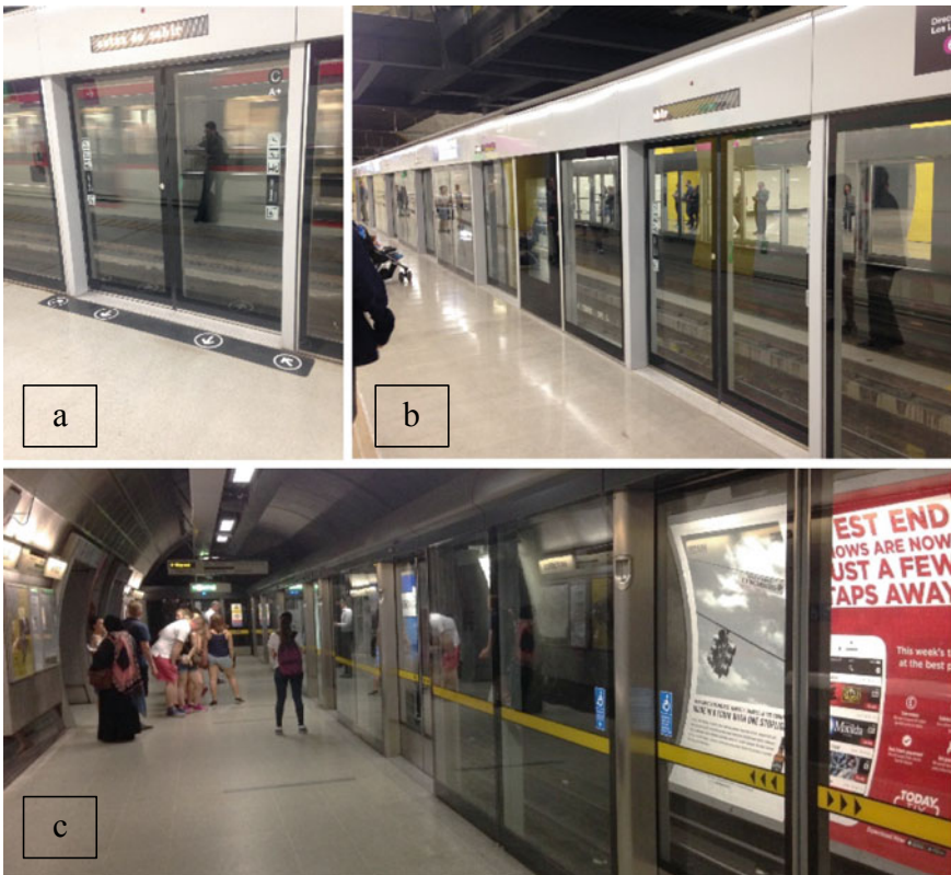
Fig. 30.1 PEDs: a Ñuble station (Metro de Santiago) with markings on the platform; b Ñuñoa station (Metro de Santiago) without markings on the platform; c Westminster station (London Underground) with markings on the platform
