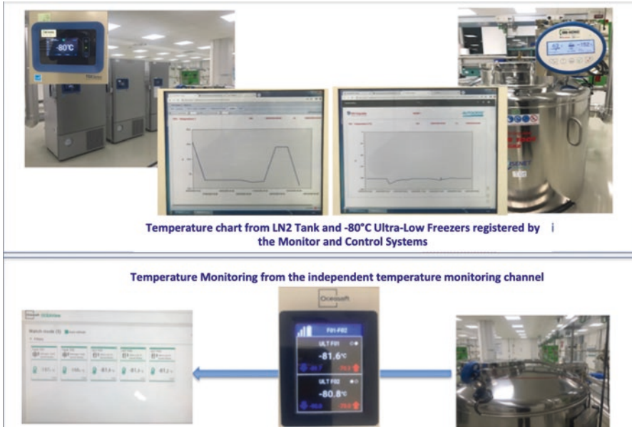
Fig. 2.12 Cold Chain monitoring and control system
