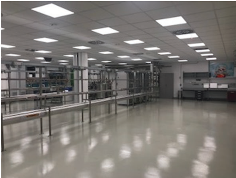
Fig. 2.3 Cryoroom Floor made with material resistant to LN2 spill
