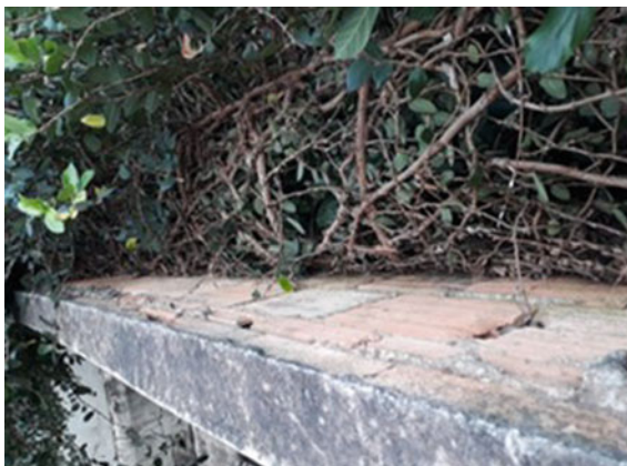
Fig. 22 Situation of the boundary wall at the back of the building
