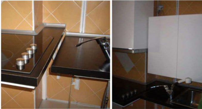
Fig. 4 Casa da D. Rosa, mechanical system of the kitchen cabinets: detail of work top in motion (author)
