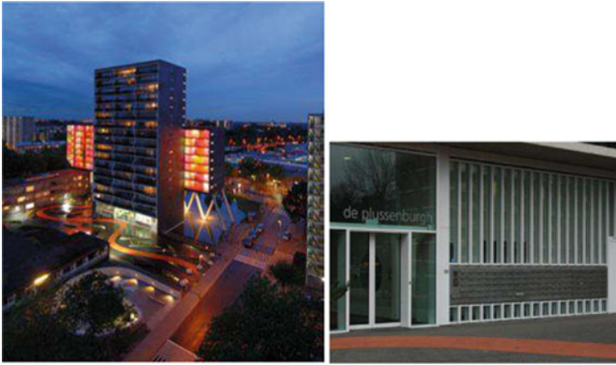
Fig. 5 Night perspectives on De Plussenburg building (Musch, Hoekstra) and main entrance (author)
