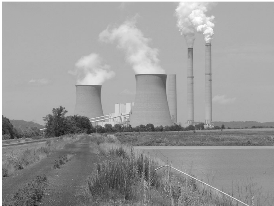
Fig. 7.13 The coal-fired Gavin Power Plant in Cheshire, Ohio https://upload.wikimedia.org/wikipedia/commons/7/75/Gavin_Plant.JPG (Wikimedia) Clouds of sulfuric acid coming from the vertical column stacks. The emissions from the Cooling Towers are just water vapor
