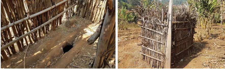
Fig. 2.8 Traditional toilet: traditional toilet enclosed with a palm front fence with wooden crossbars and squatting hole
