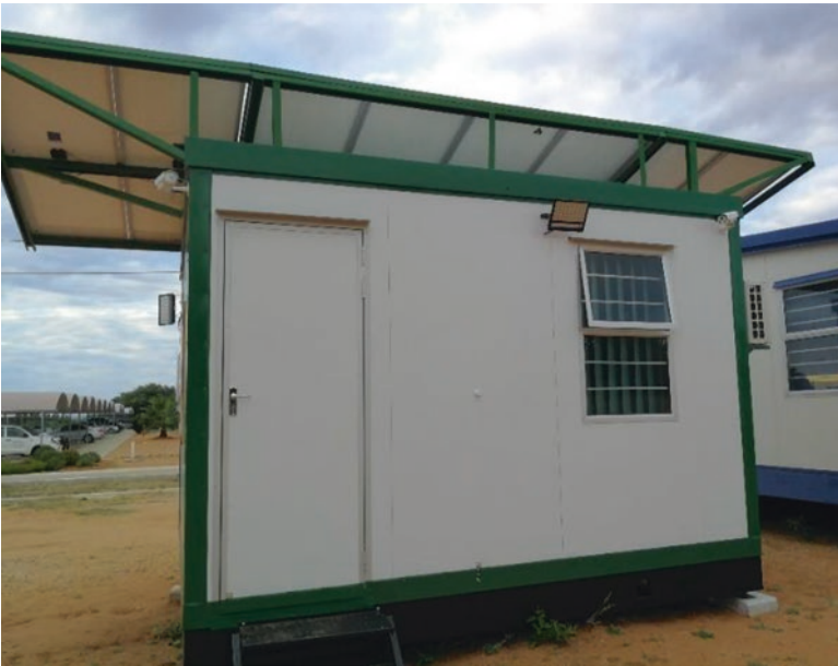
Fig. 3.20 BIUST Off-Grid secured smart house front side picture
