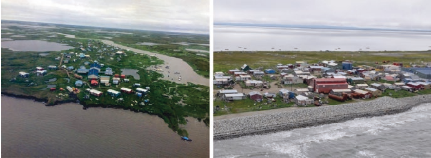
Fig. 5.3 Aerial views of Newtok, AK, where the tidal river is eroding the bank at an average rate of ~20 m/yr., and of Shishmaref, AK, where a massive revetment was constructed to prevent severe shoreline erosion associated with the loss of sea ice. (Photos from Alaska Shorezone Project, NOAA)
