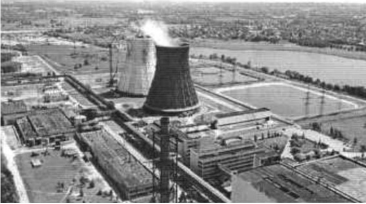
Fig. 5.3 The cooling system at the CHPP-5 (TEC-5) heating and power plant in Kharkiv, Ukraine. (Photo provided courtesy of Dr. Gennadiy K. Voronovskiy, General Director)
