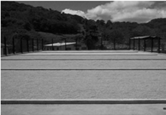
Fig. 1.13 Terrace with concrete pavement, sanitized, fenced and divided into blocks. Source: Silva et al. (2018)
