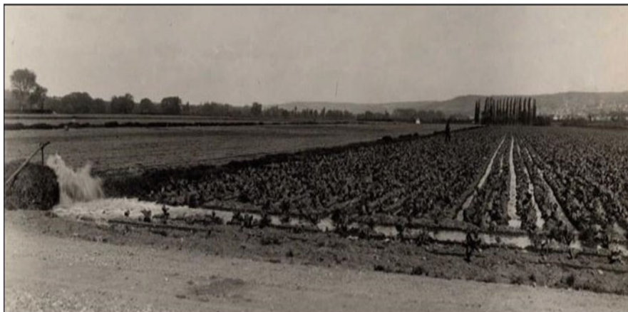
Fig. 6 Sewage farm (Credit: SIAAP)
