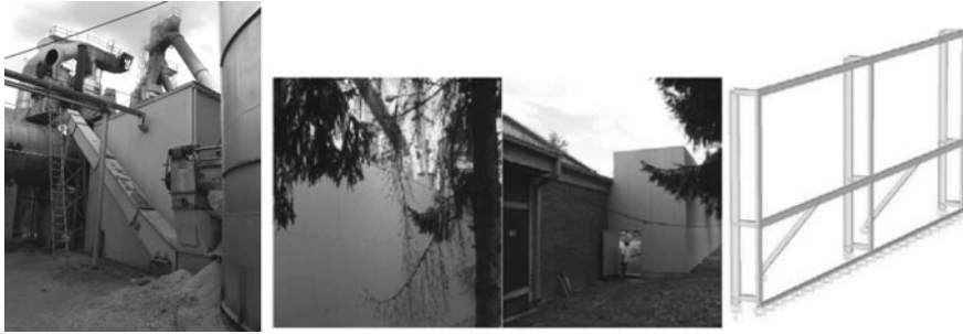
Fig. 4 Elements of the noise protection system in the “SPIK Ivanjica Fantoni Group” plywood factory
