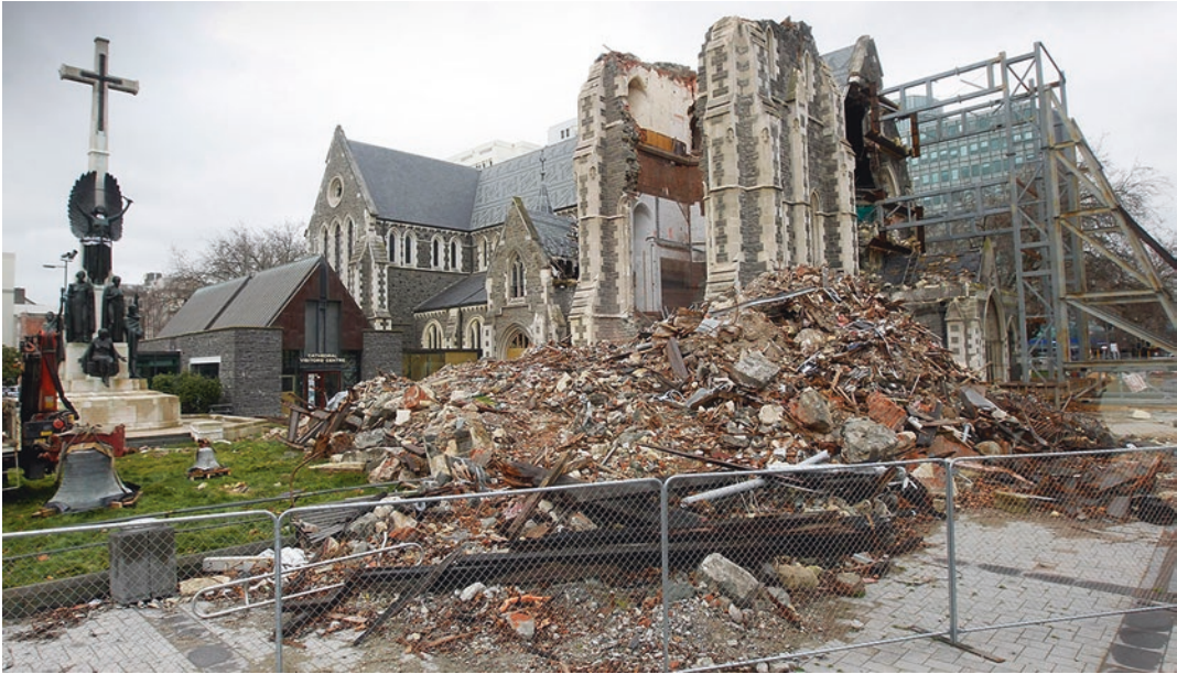
Fig. 1.2 Earthquake Christchurch 2011. (Photo by Koester 2019, CC BY 2.0)
