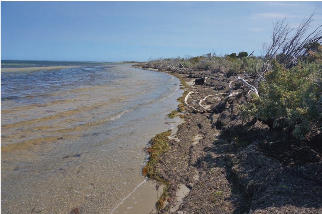
Fig. 3.2 Retreat of the shoreline at Edwards Point, Port Phillip Bay, Australia. Loss of biodiversity amongst coastlines and coastal areas due to sea level rise and changes in weather systems is already evident in many places across the world. (Photo by Author)
