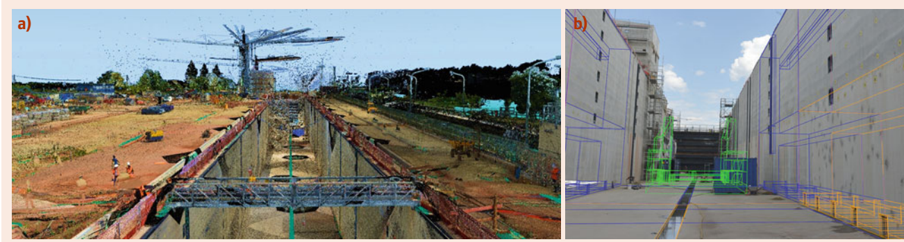
Fig. 21.2 New Trier lock: colored point cloud of a laser scanner point cloud (a), digital as-built model (b)
