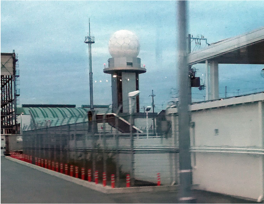
Fig. 4 Appearance of a radome at Osaka international airport
