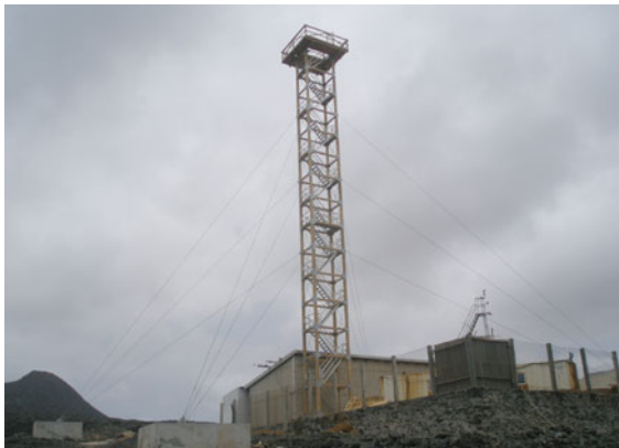
Fig. 6.7 A 30-m guyed-timber mast on the coast of São Vicente (Cape Verde Islands) (photo © Reimo Leppert, MPI-BGC)
