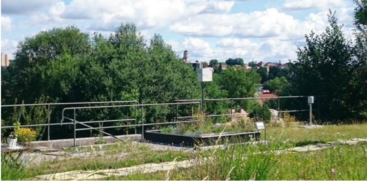
Fig. 58.6 Green roof lysimeter and climate station at the Hochschule Weihenstephan campus (photo © S. Reth)
