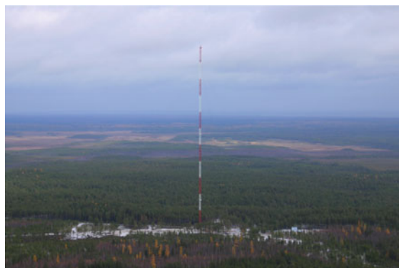
Fig. 6.16 The ZOTTO tall tower near Zotino, Central Siberia (photo © Michael Hielscher, MPI-BGC)
