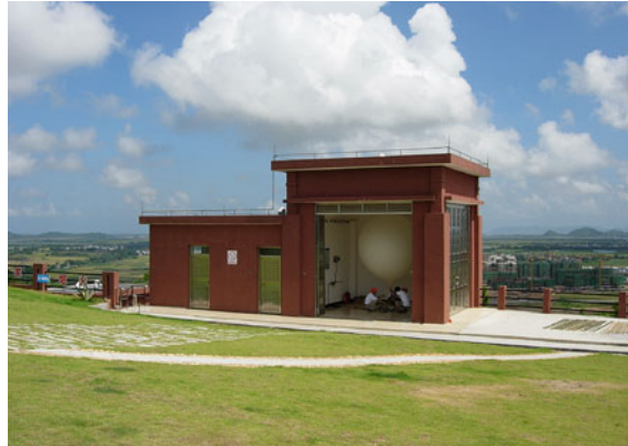
Fig. 46.9 Balloon inflation building ( right ) and hydrogen room ( left ) at the sounding station at Yangjiang China
