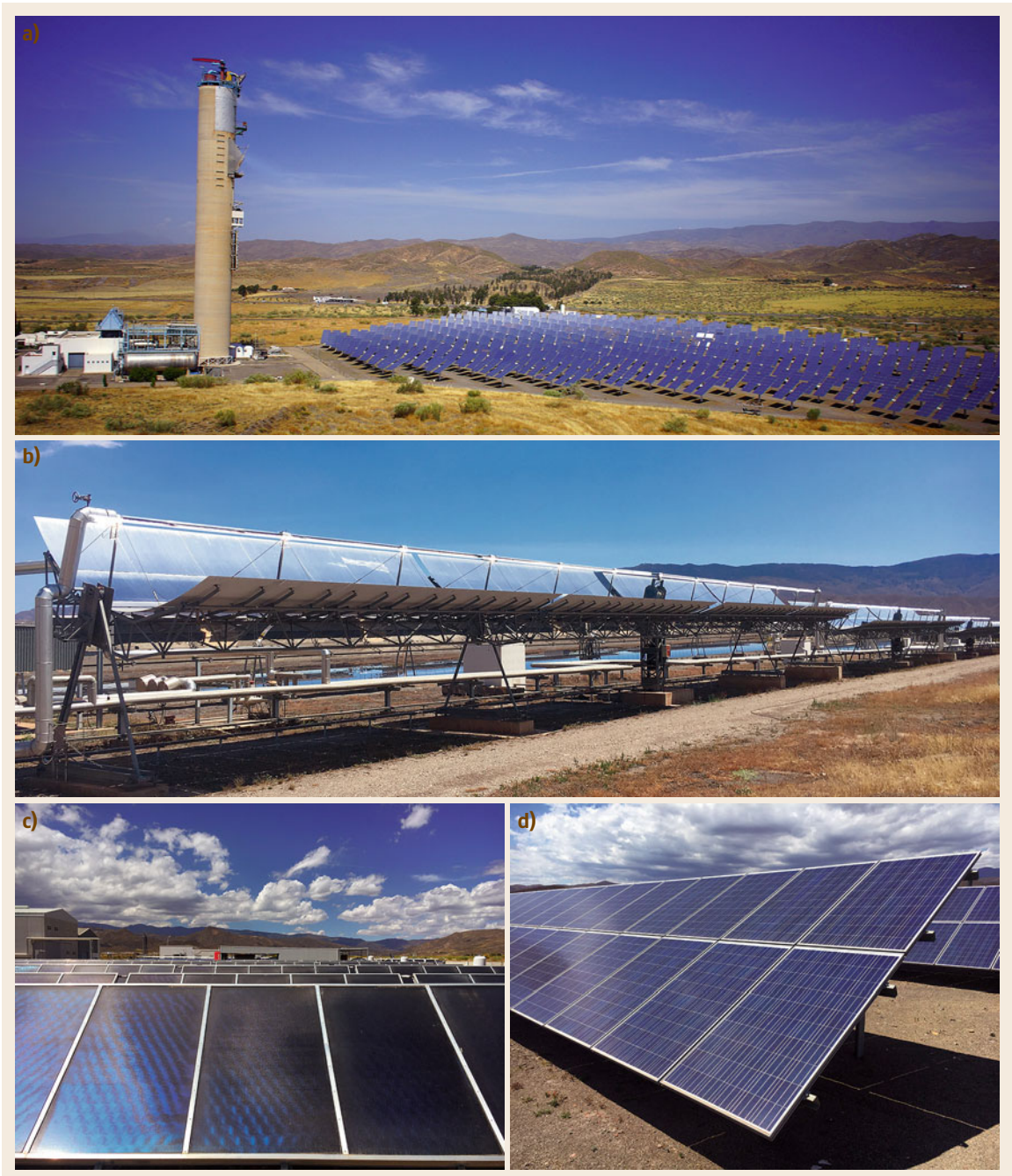
Fig. 51.1a–d Solar collectors at CIEMAT’s Plataforma Solar de Almería. (a) Tower plant CESA-1, (b) parabolic trough collector, (c) solar thermal collector, and (d) photovoltaic plant (a) photo © Christoph Prah, DLR, (b–d) photos © Stefan Wilbert, DLR
