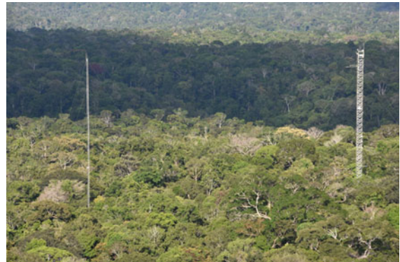
Fig. 6.29 Two 80-m masts in proximity to the ATTO tall tower (photo © Martin Hertel, MPI-BGC)
