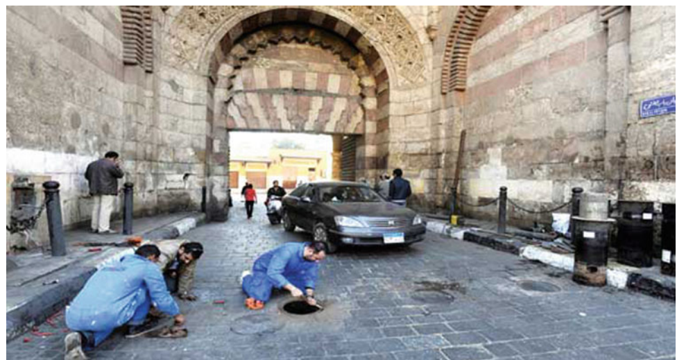
Fig. 6 Maintenance of Al-Moez Street electronic gates. http://gate.ahram.org.eg
