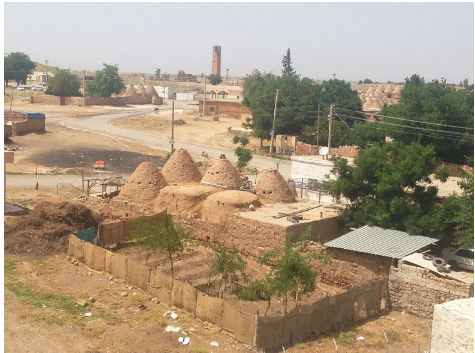
Fig. 4 A group of Harran Houses (Özdemir and Çetiner Özdemir 2014) Traditional Harran Houses have domes which are covered with brick due to lack of wood. In addition, there were quite abundant brick material that are found in ruins of Harran
