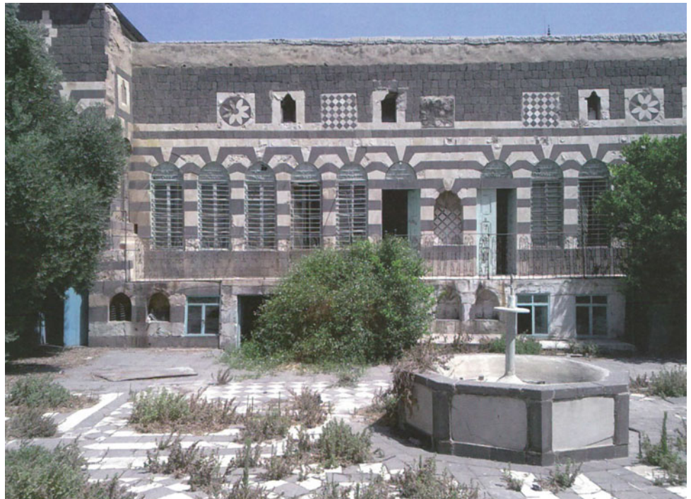
Fig. 16 Windows latticework in Homs Courtyard house: (Al Dandashi 2013)
