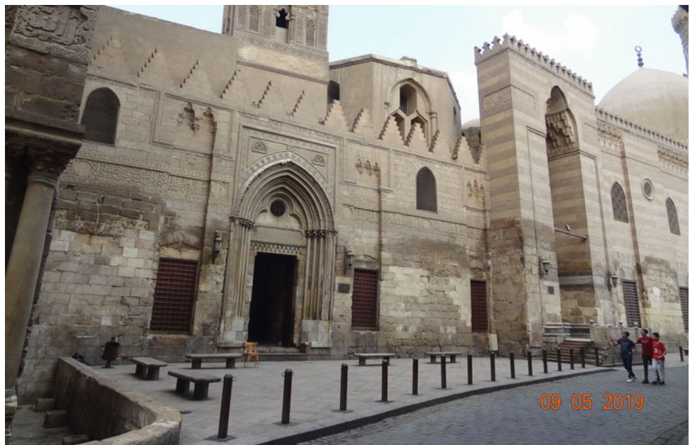
Fig. 4 Distribution of landscaping elements before historic buildings. (Photo by the author)
