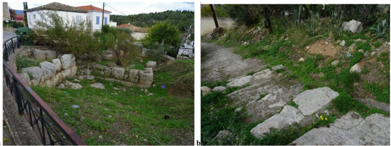
Fig. 3 a Wall and adjoining tower inside an impromptu fenced enclosure. b Remain of the wall crossing a street
