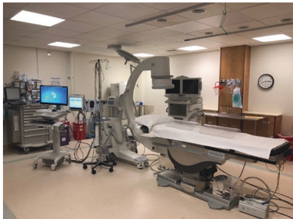
Fig. 27.1 Image of EP room. Procedure rooms vary widely in layout. This room poses problems for the anesthesia team because the X-ray machine is placed near the patient's head, away from the oxygen and suction lines, and there is no readily available anesthesia machine
