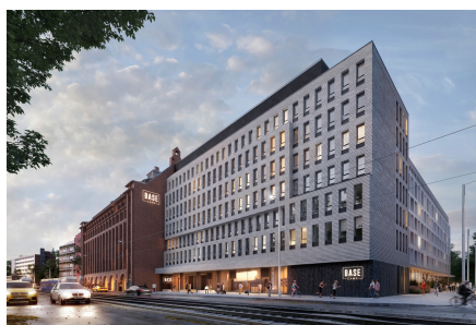
Fig. 1. (left) Basecamp dormitory complex (designed by Grupa 5 Architekci) - adaptive-reuse and extension of Mamut bakery in Wrocław planned to be realised in 2020 (PL). On the left: ceramic-cladded floor storage building adapted for main entrance zone and dormitories, on the right: new wing of the Basecamp dormitory (visualisation by Grupa 5 Architekci [15]).
