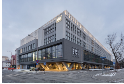
Fig. 2. (right) Basecamp dormitory complex (designed by Grupa 5 Architekci) realised in Łódź in 2017 – adaptive-reuse of Dzielowa Printing House (PL) (photo by Grupa 5 Architekci [16]).
