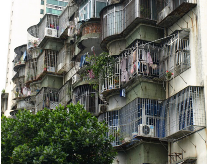
Fig. 8. Balcony grids as additional protection against burglary (Shenzhen, China, photograph by the author).
