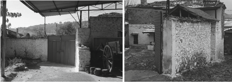
Fig. 3. Entrance doors and gate, from outside and from inside. The materials used are a whitewashed wall made of stone, a roof over a door made of wood, a balustrade of a terrace made of perforated brick. The door and entrance gate are made of steel. Back walls of the house, view from the streets. The ground floor is heavily built-up. There are practically no windows on the ground floor. From this side the house is a closed fortress, fenced with a 200 cm high stone wall and does not show its internal composition. Photos: Alicja Maciejko, 2018.
