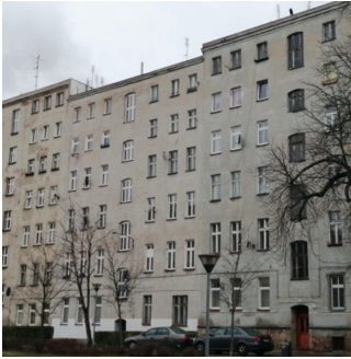
Fig. 3. Elevations of tenement houses from the 19 th /20 th century on the courtyard side without balconies (photograph by the author).
