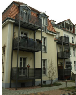
Fig. 4. Contemporary balconies of steel construction at a historic building (photograph by the author).
