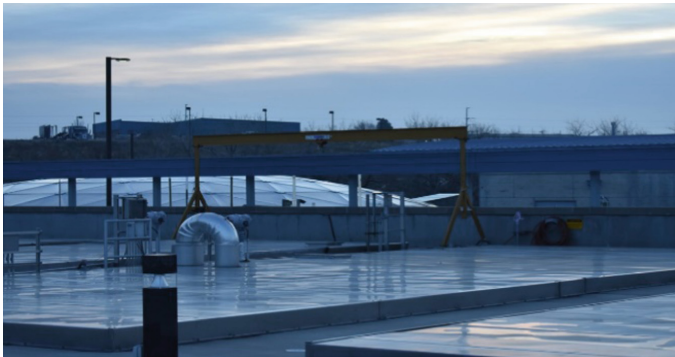
Fig. 3. Gantry used to move some panels.
