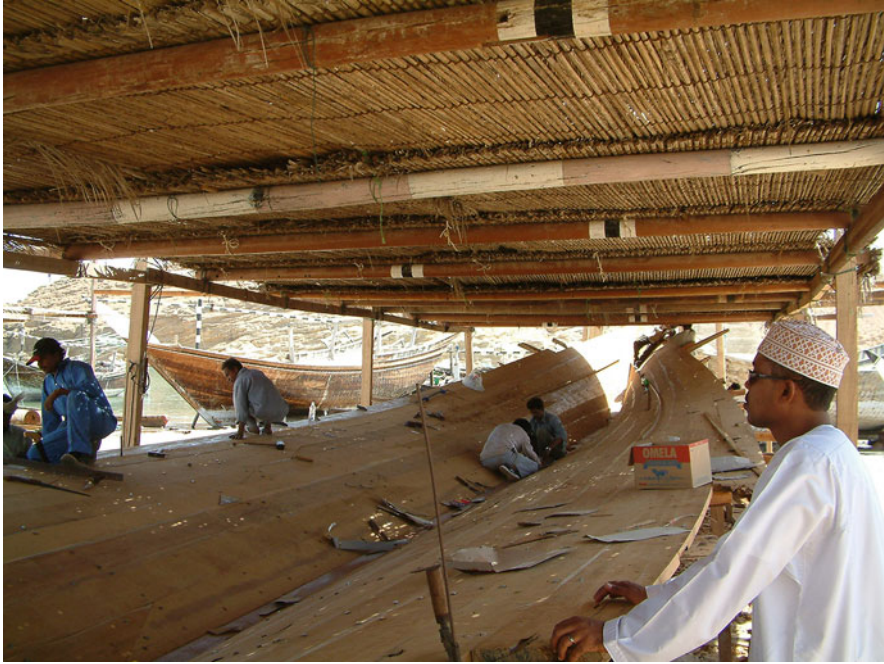
Fig. 2 Shū'ī under construction, inside, Sur 2003, courtesy of Piotr Dziamski, Poland
