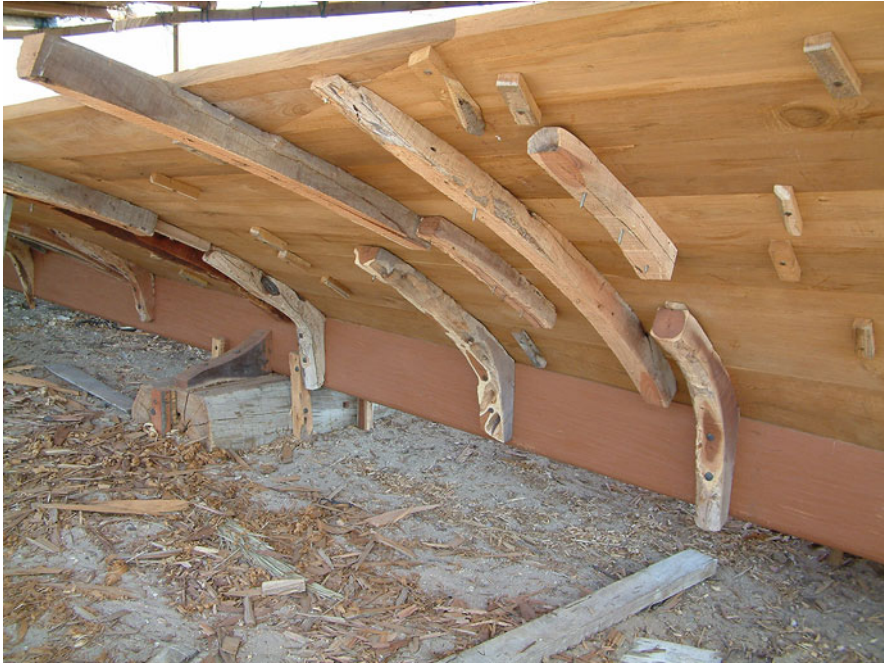
Fig. 3 Shūṛ under construction, outside, Sur 2003, courtesy of Piotr Dziamski, Poland
