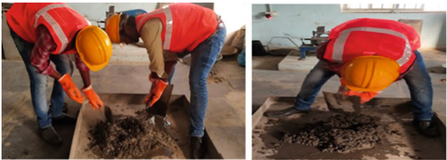
Fig. 2 Preparation of concrete mix
