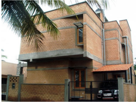
Fig. 1 Case study building
