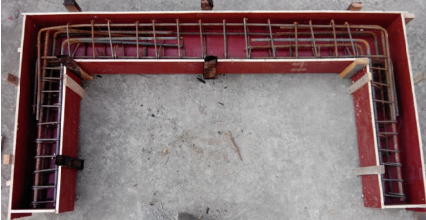
Fig. 2 Reinforcement placement in the formwork cage
