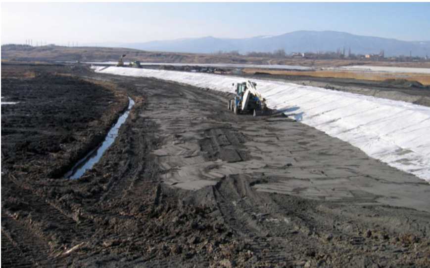
Fig. 6 Construction of a new earth dike
