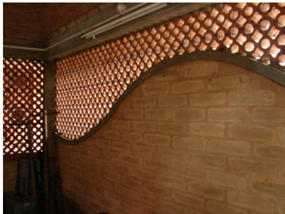
Fig. 1 The interior of a stabilized soil block building on the campus of Indian Institute of Science, Bangalore
