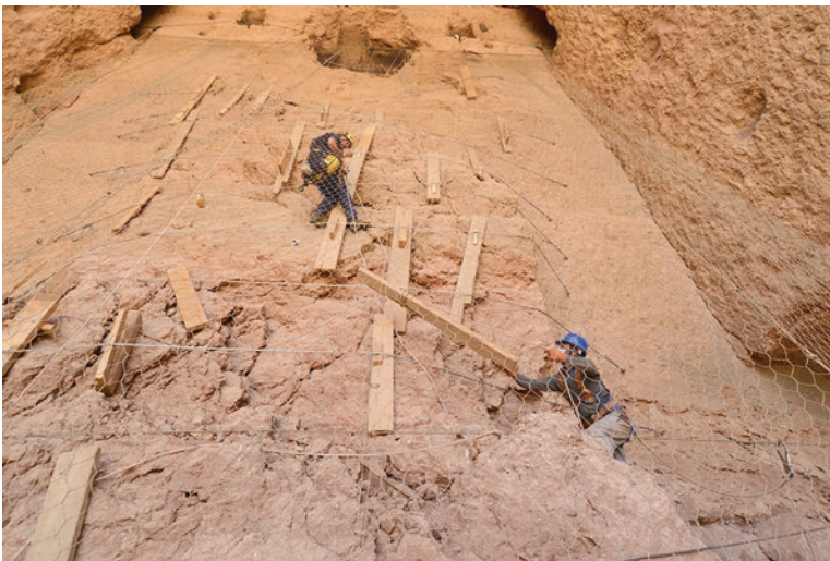
Photo 11 Western Buddha niche, September 2017: Prestabilisation measures on Western Buddha rear face, former head area (BRR-team Klaus Vogt und Haji Hossein). (© Bert Praxenthaler)
