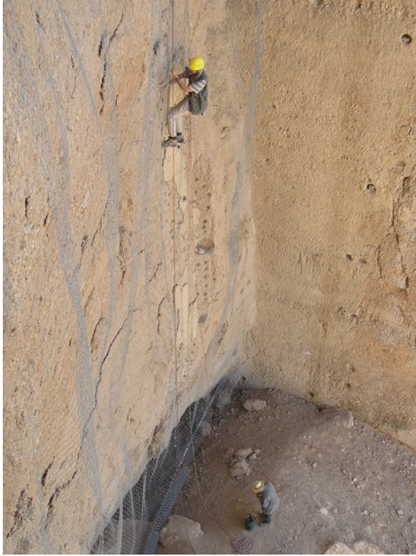
Photo 4 Eastern Buddha, July 2004: Emergency safeguarding of original fragments of clay plaster at the rear face of the Eastern Buddha. (© Bert Praxenthaler)
