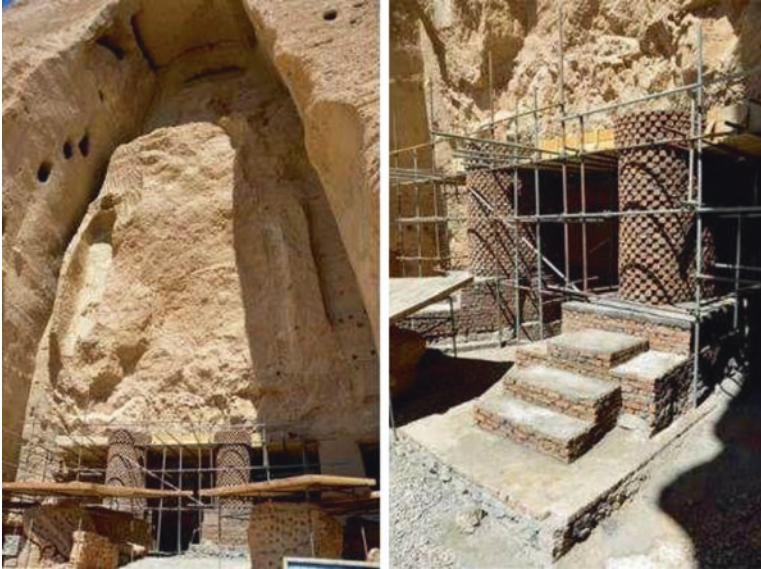
Fig. 3 Situation at the niche of the Eastern “Small” 38 m Buddha as of December 2013, pillars made of reinforced concrete constructed by restoration team of Technical University of Munich. (© UNESCO)
