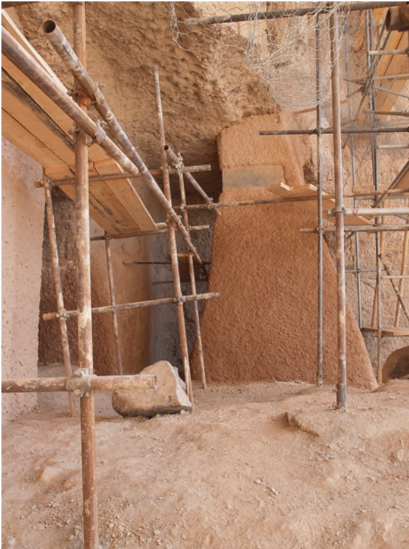
Photo 7 Eastern Buddha, September 2009: reconstruction of cave walls and a pillar at the lower gallery by Erwin Emmerlin, Edwin Fecker and Sekandar Seradj. (© Bert Praxenthaler)
