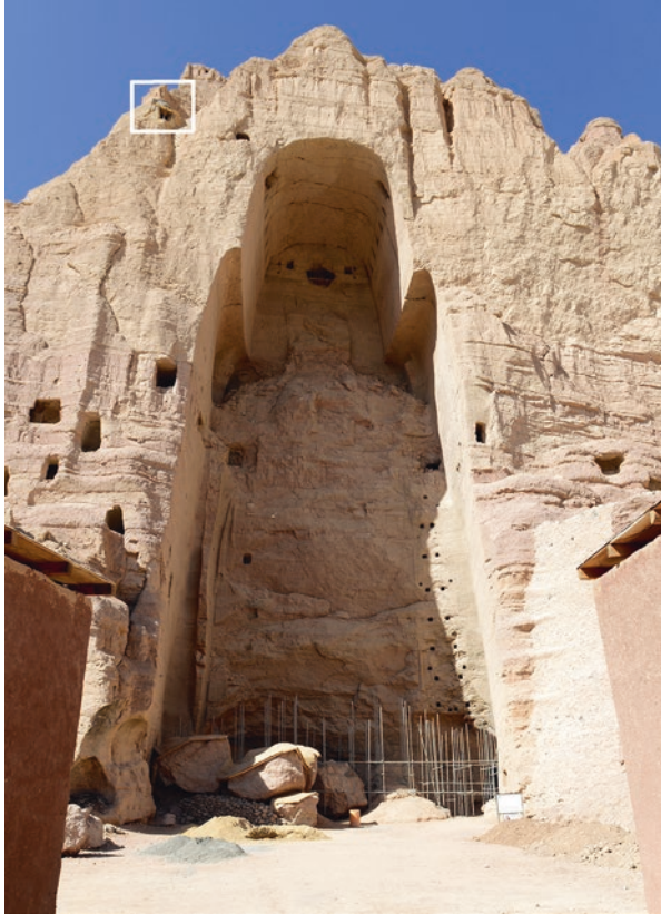
Photo 8 Western Buddha, October 2013: Safeguarding the upper access to the top of the Buddha (marked in white, top left). (© Bert Praxenthaler)
