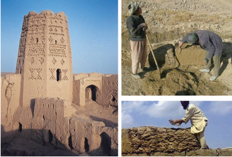
Fig. 7 (Left) Traditional “Qala” house in Afghanistan with octagonal tower, decorations carved into the soft wall during construction. (Right) Construction process of a traditional “pachsa” cob wall in line segments with finish of fine “kaghel” plaster. (© P. Smars/RWTHAcdc)
