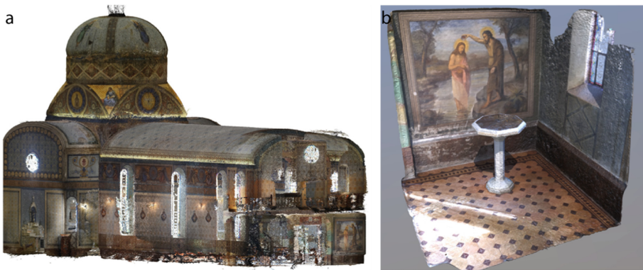
Fig. 5. (a) Negative point cloud from interior of St. Peter Chapel, and (b) TIN mesh of the Baptistry
