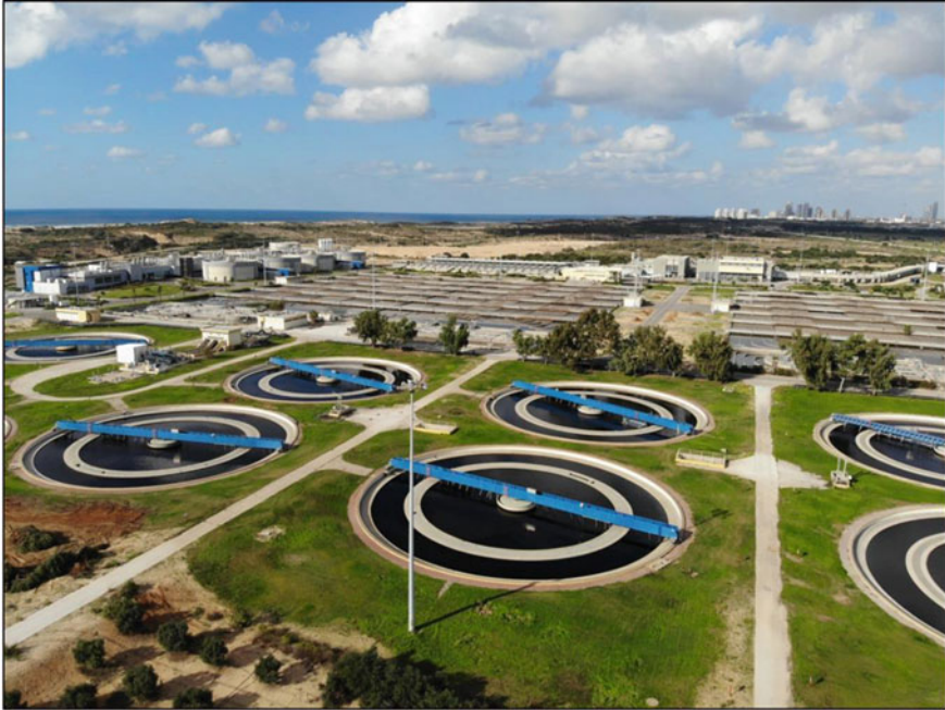
Fig. 2 Shafdan WWTP (partial view). The raw sewage inlet pipe, the biological reactors and the clarifiers can be seen from back to front
