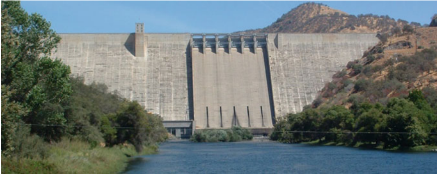
Fig. 1 Downstream view of Pine Flat Dam [2]
