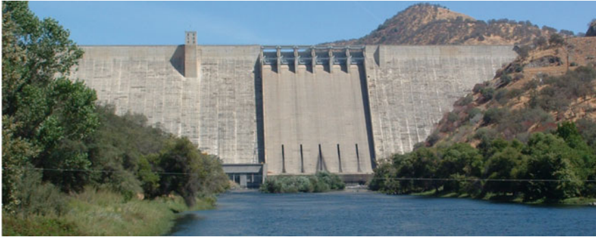
Fig. 1 Downstream view of pine flat dam
