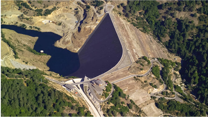
Fig. 1 Menta embankment dam
