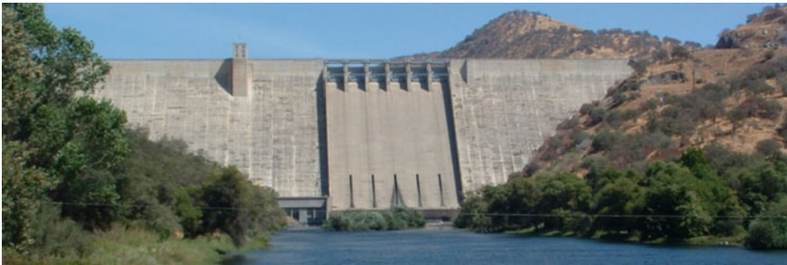
Fig. 2 Downstream view of Pine Flat Dam
