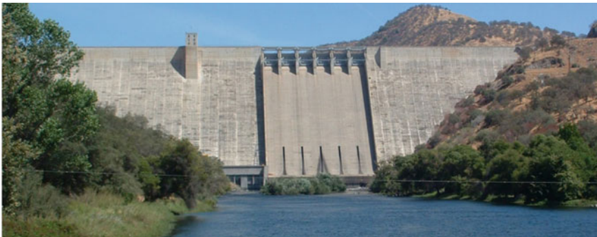
Fig. 2 Downstream view of Pine Flat Dam [15]
