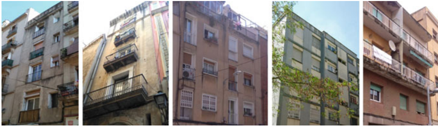
Fig. 17 Buildings with cornices, balconies and sills in poor condition
