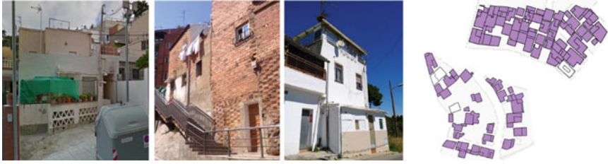
Fig. 8 Examples of Type 3 buildings in Torre Baró and Vallbona
