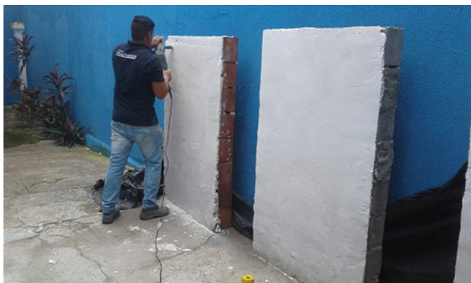
Fig. 12 Cut of the coating using a cup saw
