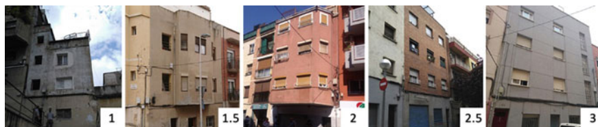
Fig. 3 Need for refurbishment rating: 1 urgent, 1.5 high, 2 necessary, 2.5 low and 3 very low
