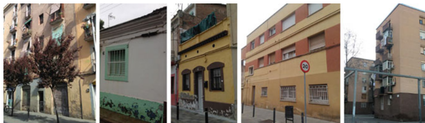
Fig. 16 Cases of rising damp due to capillarity
