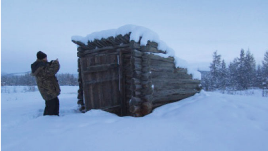
Fig. 14.10 More than 100 years old cellar at Oymiakon, Sakha Republic where recent fall storm-flooding event and filling by ice
