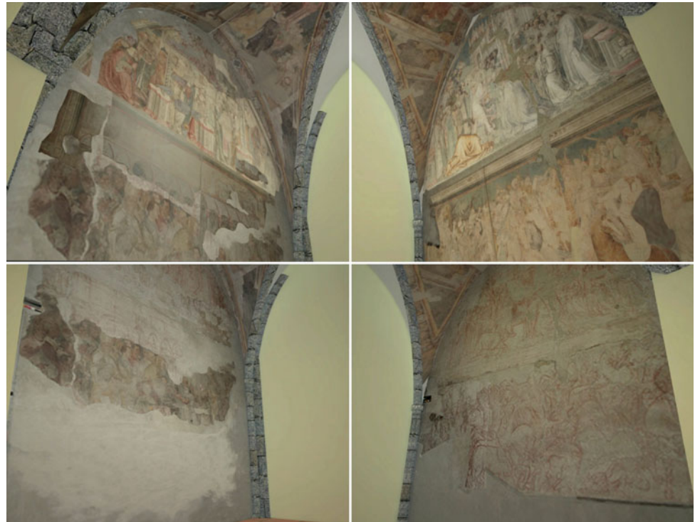
Fig. 5 Three-dimensional reconstruction of the current configuration (below) and original configuration (above) of the frescoes on the side walls of the Chapel of the Crucifix
