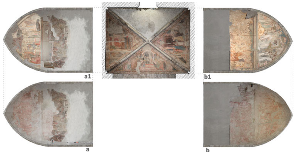
Fig. 6 Plan of the ceiling with rabattment of the side views of the Chapel of the Crucifix in the current configuration (a and b) and the virtual reconstruction (a1 and b1)
