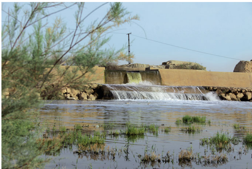
Fig. 5.10 Jondij Old Dam
