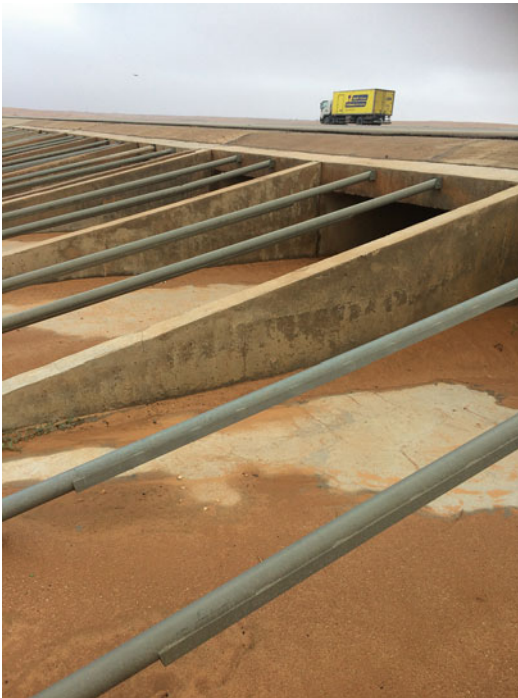
Fig. 25.11 Example of dyke and culvert to manage potential wadi runoff (Source: Halim Maamari)
