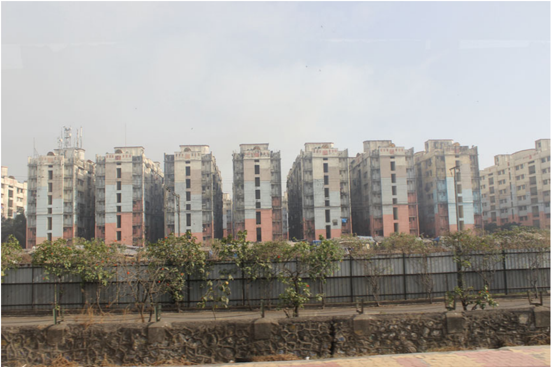
Fig. 7.5 Extreme compaction in multi-storey housing after slum rehabilitation (Source: Peter Morgenstein)
