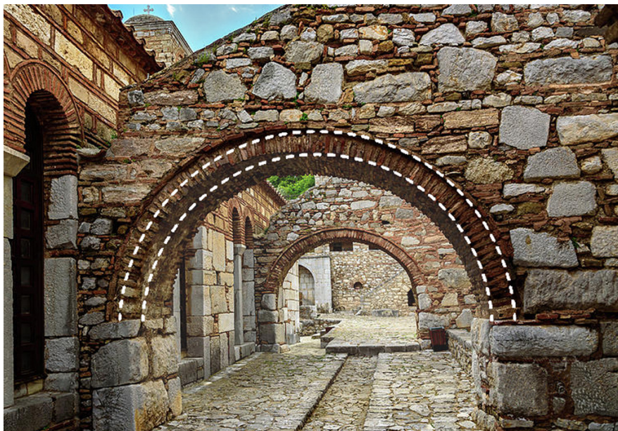
Fig. 27.1 Monastery Of Hosios Loukas in Greece. In dashed white lines the circular arc with nominal thickness and radius.
