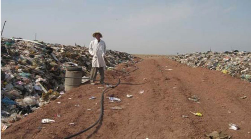
Fig. 2.6 Bioreactor landfill using leachate recirculation
