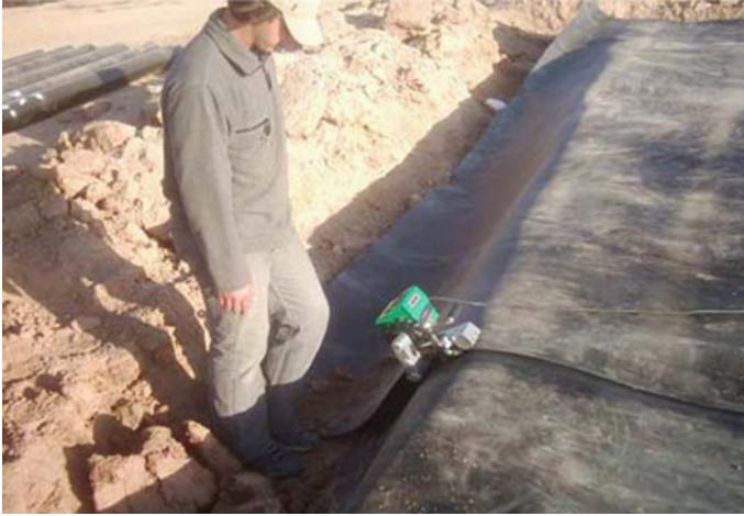
Fig. 2.19 Installation of a flexible membrane liner
