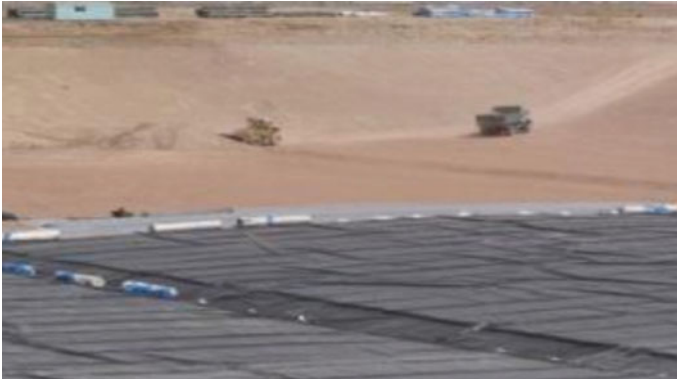
Fig. 2.32 Application of geomembrane in landfill
