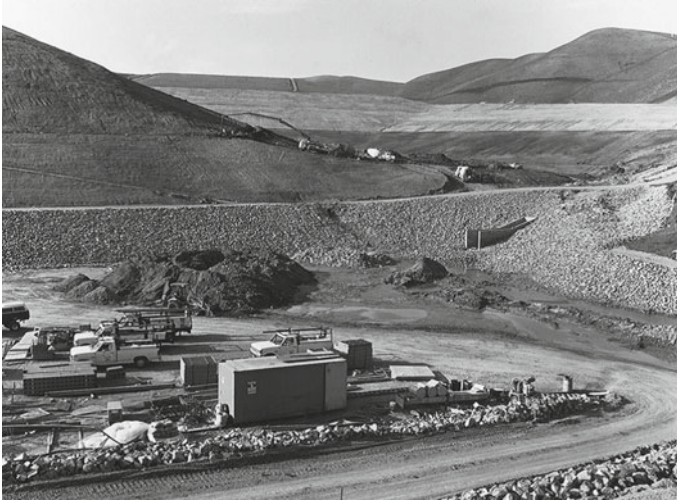
Fig. 2.28 View of large stormwater retention/storage basin at a large landfill. The size of the basin can be estimated from the size of the vehicles parked at the bottom of the basin
