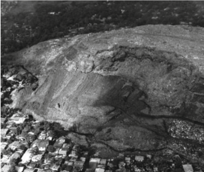
Fig. 2.7 Landfill slope failure
