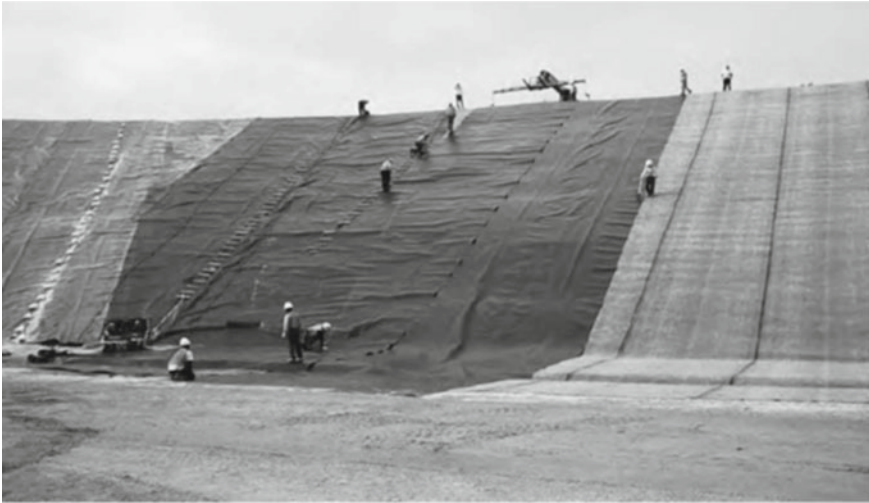
Fig. 3.11 Synthetic liner on the slope, ready for earth cover
