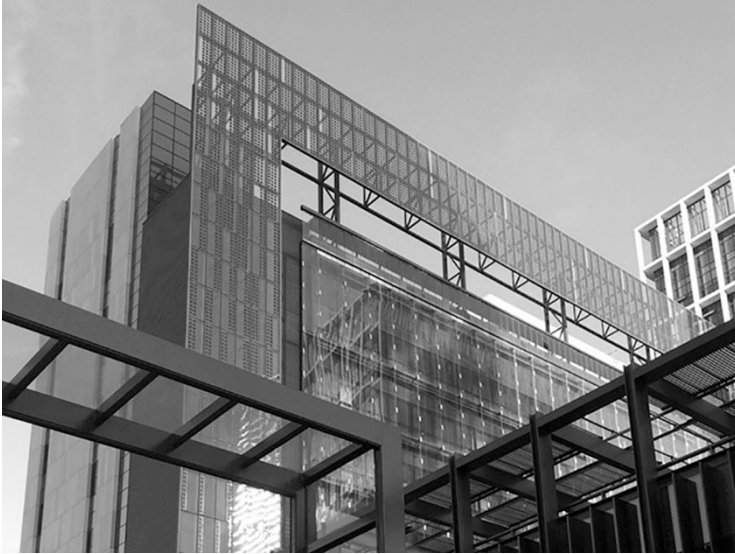
Fig. 5 TEDA Administrative Commission office building with BIPV panel. Source: AECOM
