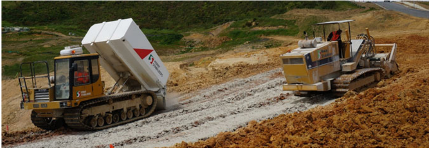
Fig. 1 Example of low ground pressure spreader and stabilizer undertaking fill drying
