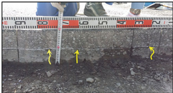
Fig. 4 Cut section of asphalt pavement (another expressway)
