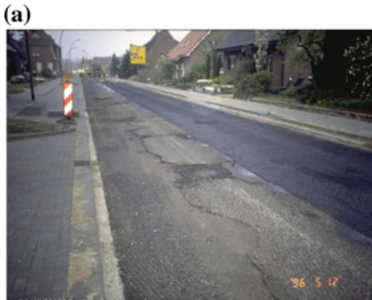
Fig. 3 a Condition after milling in May 1996, b Condition in March 2013
