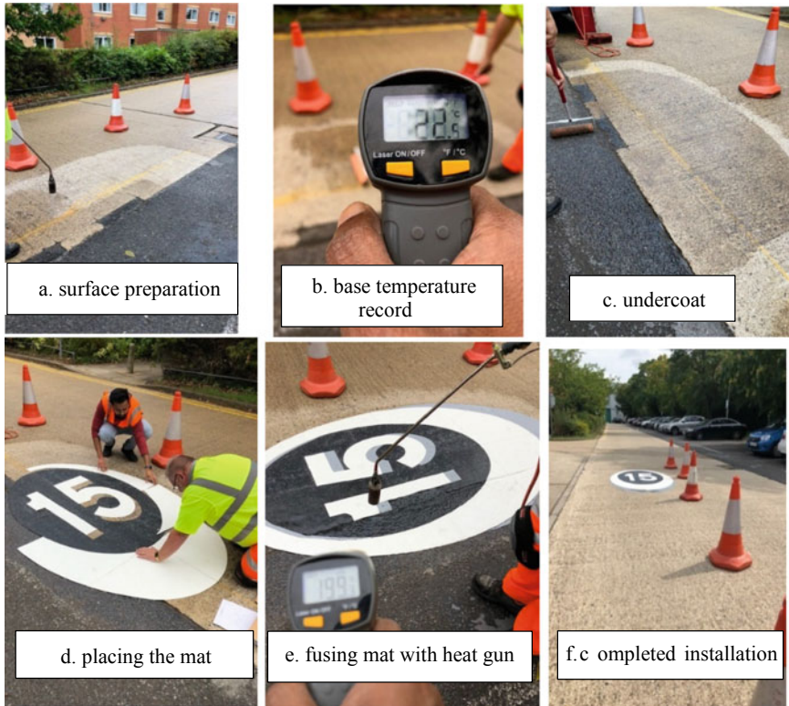
Fig. 2 3D preformed marking installation procedure
