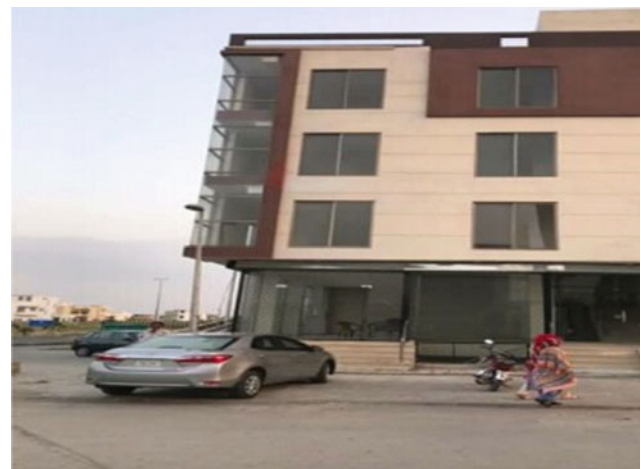
Fig. 1 Commercial building on site
