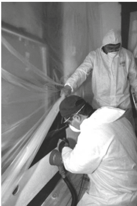
Fig. 3 CPS Attic cellulose insulation on top of existing fiberglass insulation (Danner 2012)
