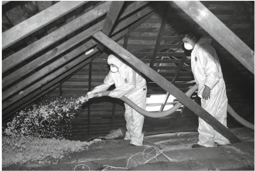
Fig. 2 CPS Wall Insulation installed at a residence's home
