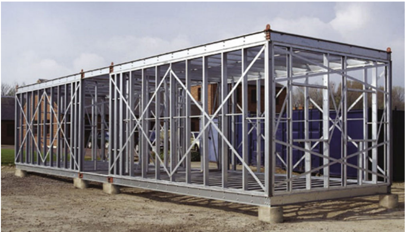
Fig. 1 Modules selected for the case study project construction
