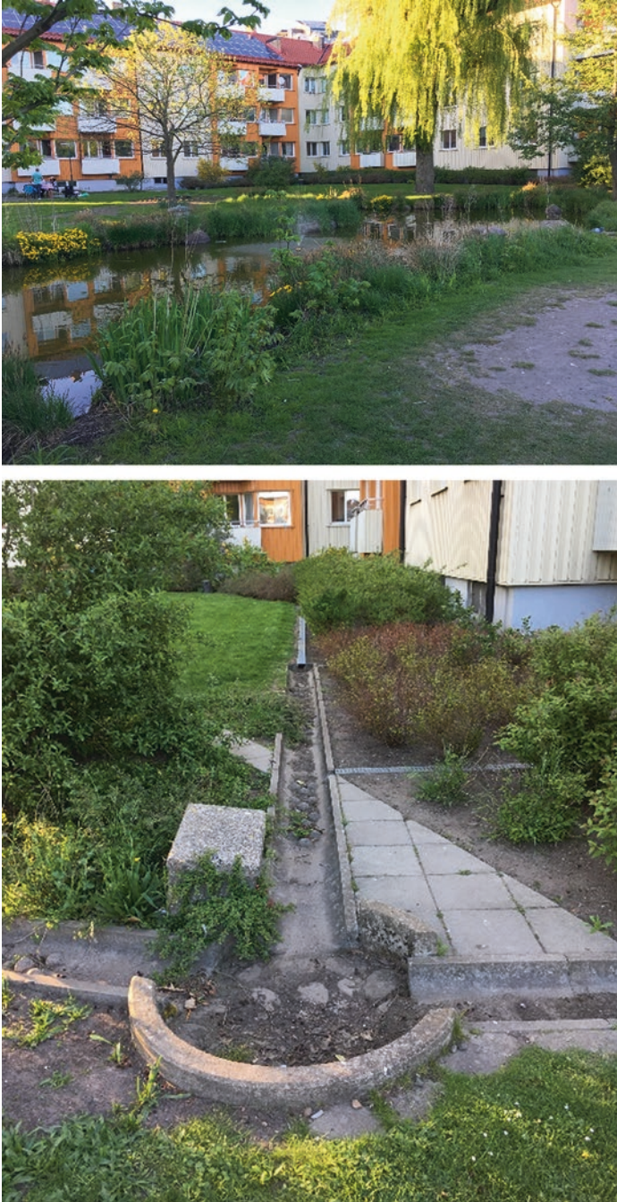
Fig. 5 Open stormwater drainage in Augustenborg, a social housing area in Malmö, Sweden (photo by Åse Johannessen)
