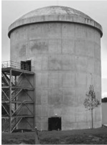
Fig. 2. EDF Vercors 1:3 scale mock-up for NPP containment ageing study
