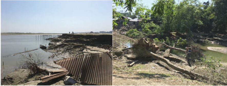
Fig. 3 Some pictures of losses and damages of 2017 flood
