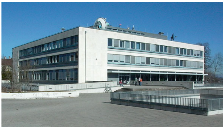
Fig. 3 Present look of the building at Sidlerstrasse 5 (photo and ©: Chr. Schläppi)
