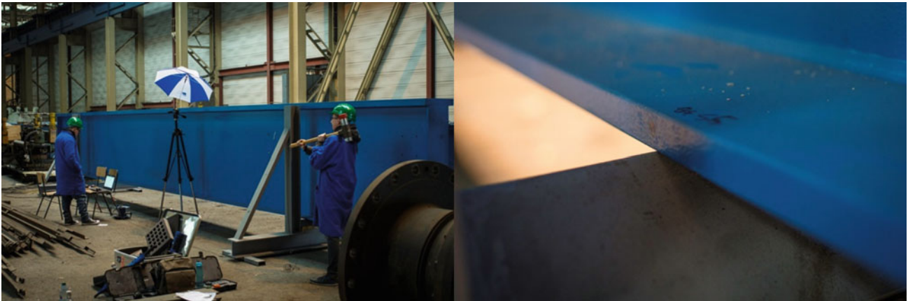
Fig. 37.4 Left – runway beam under study. Engineers and equipment depicted for scale. Right – detail of the beam supported on L-shaped profiles around DOF 55
