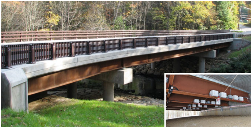
Fig. 2.4 Powder Mill Bridge (PMB) over the Ware River in Barre, MA
