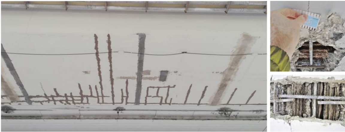
Fig. 19.5 Visual inspection campaign carried out on the bridge
