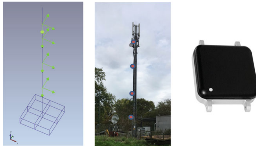
Fig. 3.2 Left. Acquisition Scheme using OPAL system. Centre. OPALs installed in monopole. Right. OPAL sensor
