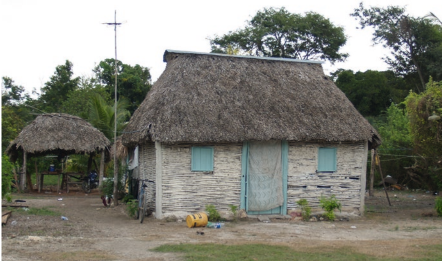
Fig. 30.6 An atypical residence for the upriver area, but common among Mayan rural communities, crafted from woven wood, covered with wattle and daub spackle, and crowned by a perishable, huano palm ( Sabal spp.) thatched roof
