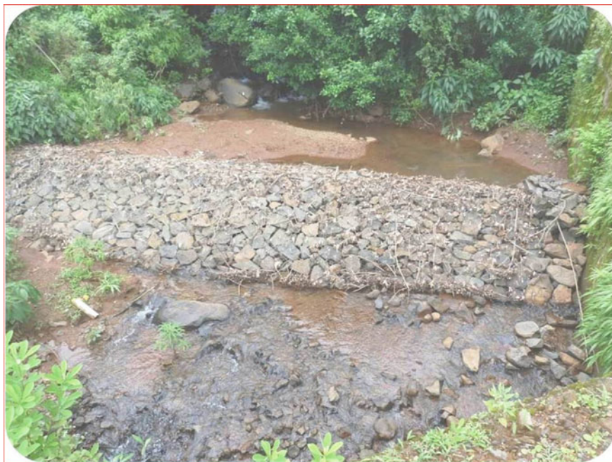
Plate 3.2 Loose boulder structure at Undri village
