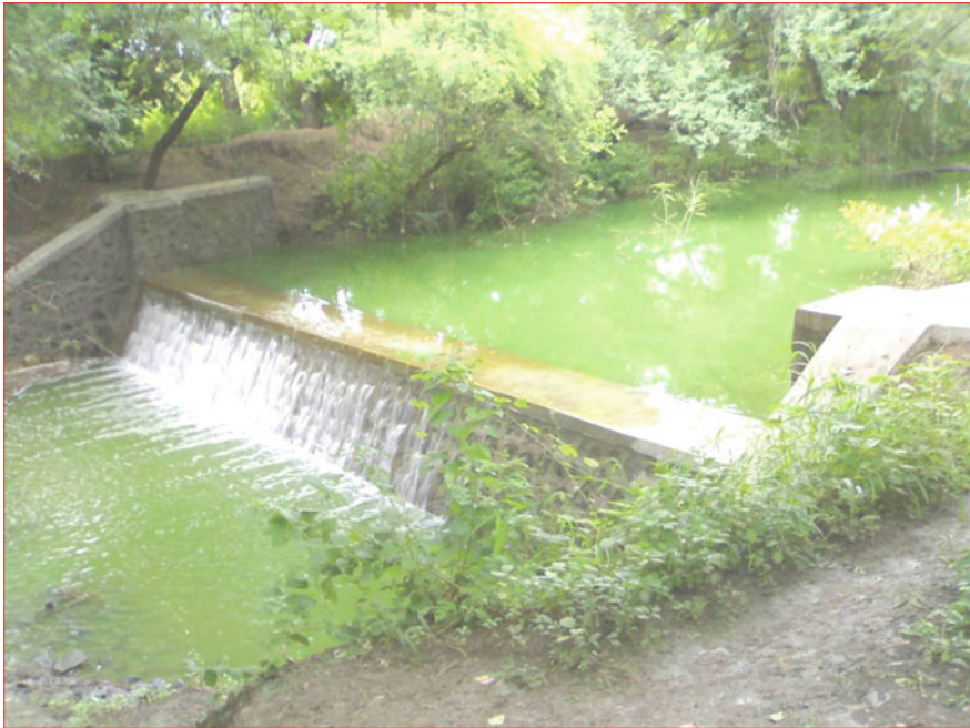
Plate 3.1 Cement nala bund at Atali village
